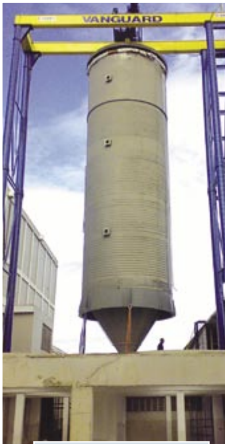
The 21-metre-long tank is lowered into final position.
