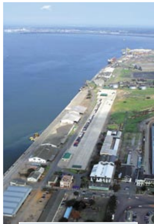
An aerial view of the Maputo Car Terminal.
